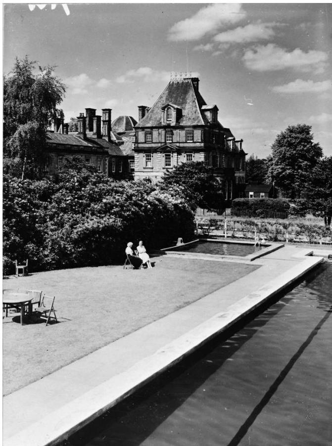
Swimming pool in 1959, during ICI's ownership
