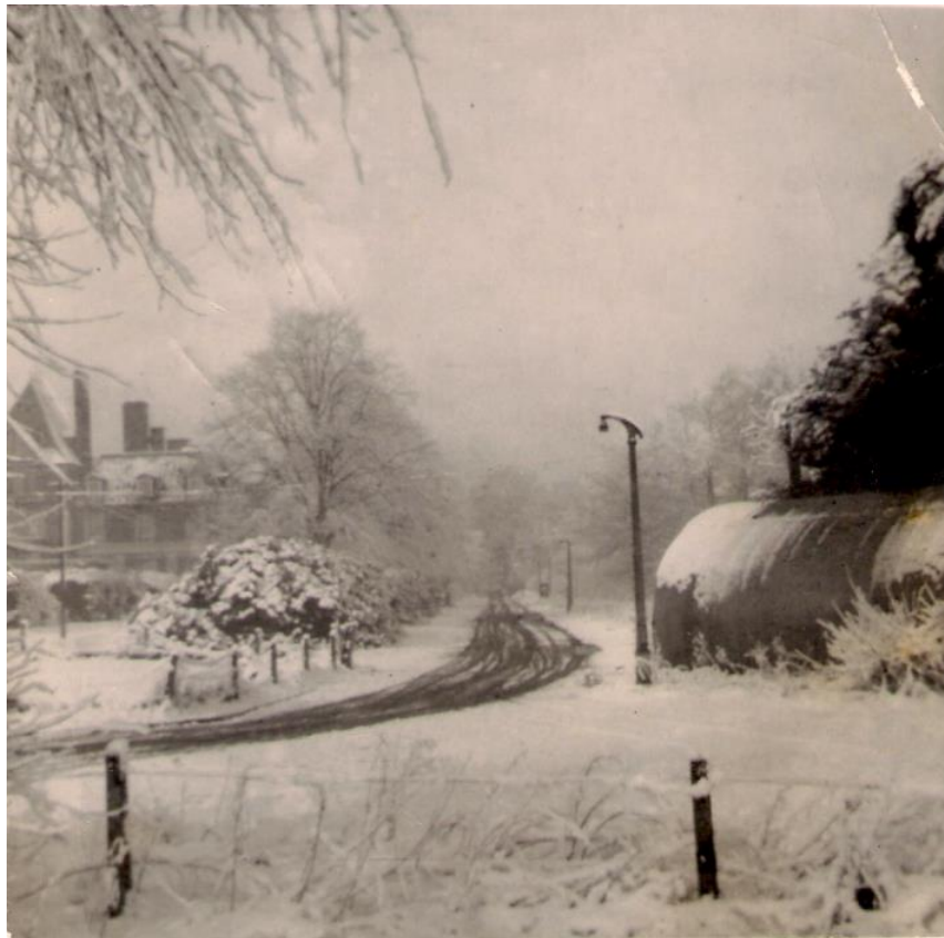
View from the Campbell's garden – 100 East Park (early to mid 1960's) (the entrance to the present Rangers' compound is opposite the lamp post)
