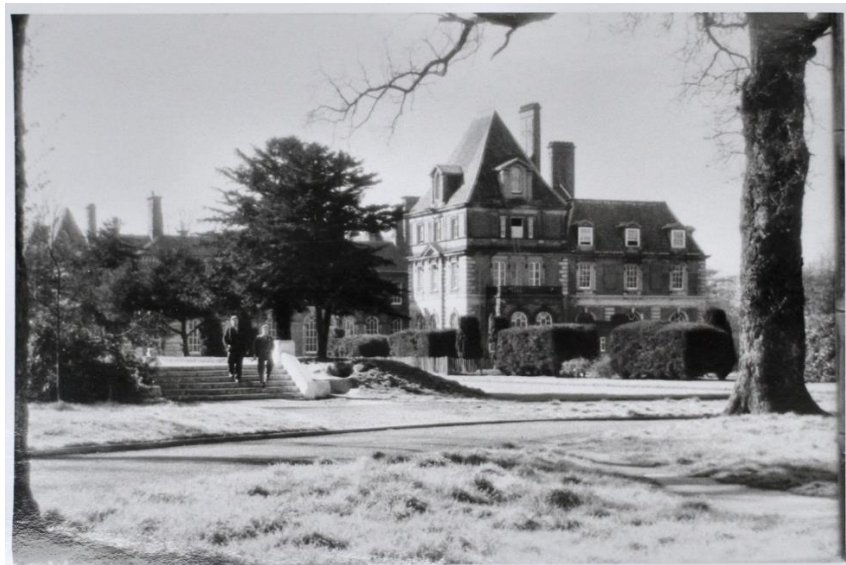
View of the east side of the hall
