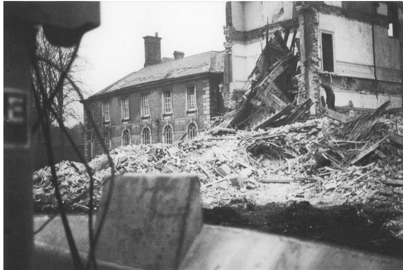
Demolition of Marbury Hall
