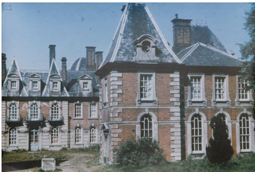
View of the south side of the hall
