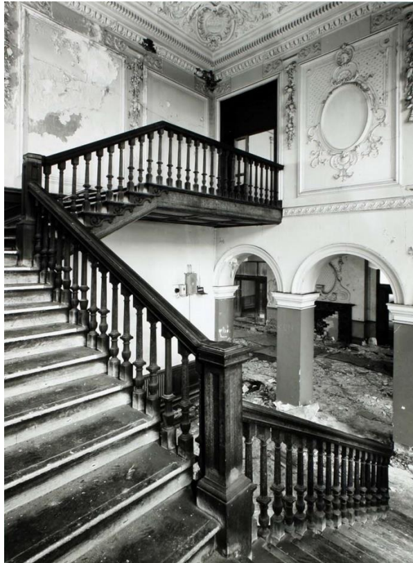
Main staircase looking towards hall
