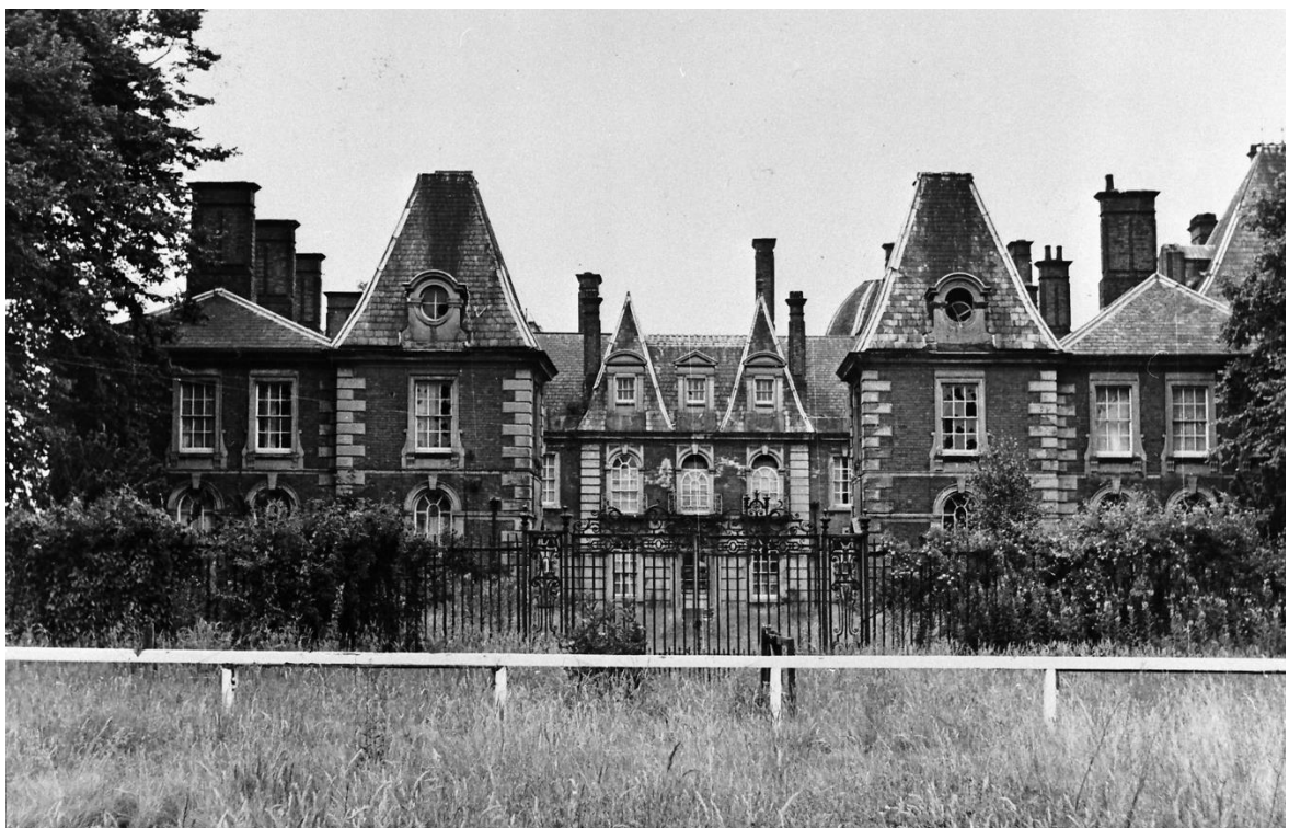
Neglected and no longer weather-tight
